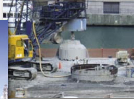
Case Foundation used a 114" Center Rock L.P. Drill system to drill 48 holes, 35 feet in depth, for the foundation caissons of the Trump Tower under construction in Chicago.
