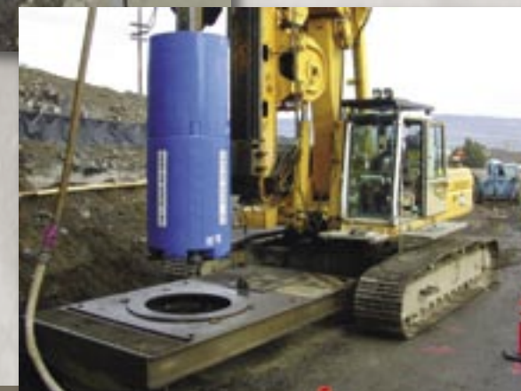
Our L.P. drills are frequently used to cut foundation holes for highway overpasses and related support construction. Here a contractor uses a 48" Center Rock L.P. Drill to cut support holes for a new overpass.
